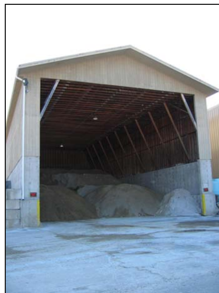
Salt Storage Facility
