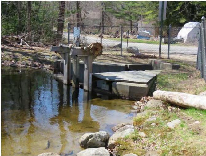
White Oak Pond dam at elevated average water level of 1.9 ft.
